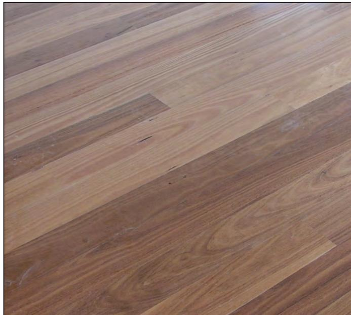
*Engineered floor laid on acoustic underlay*
